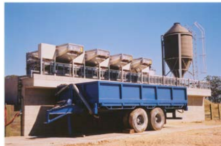
General Arrangement of multiple V-FOLD™ filters
