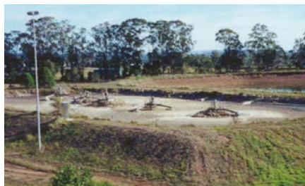
Aeration lagoon (6 M litre)
